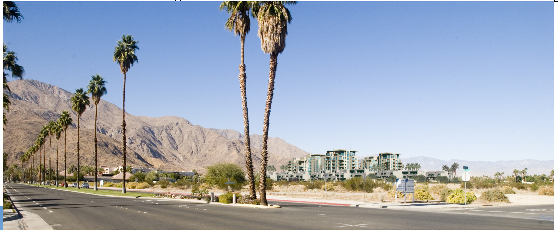
E. TAHQUITZ CANYON ROAD AT N HERMOSA DRIVE LOOKING NORTHWEST
